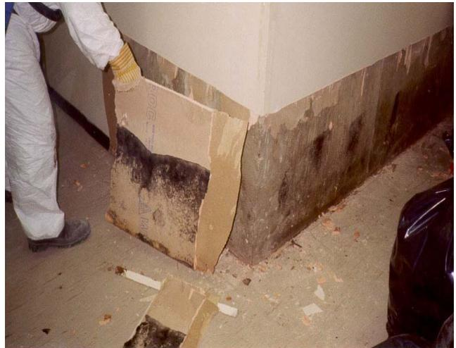
**Example of mould growth on the inside of a wall after a flood.**
